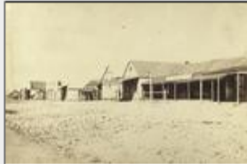
Buildings in Christoe Street, Copperfield, 1876
